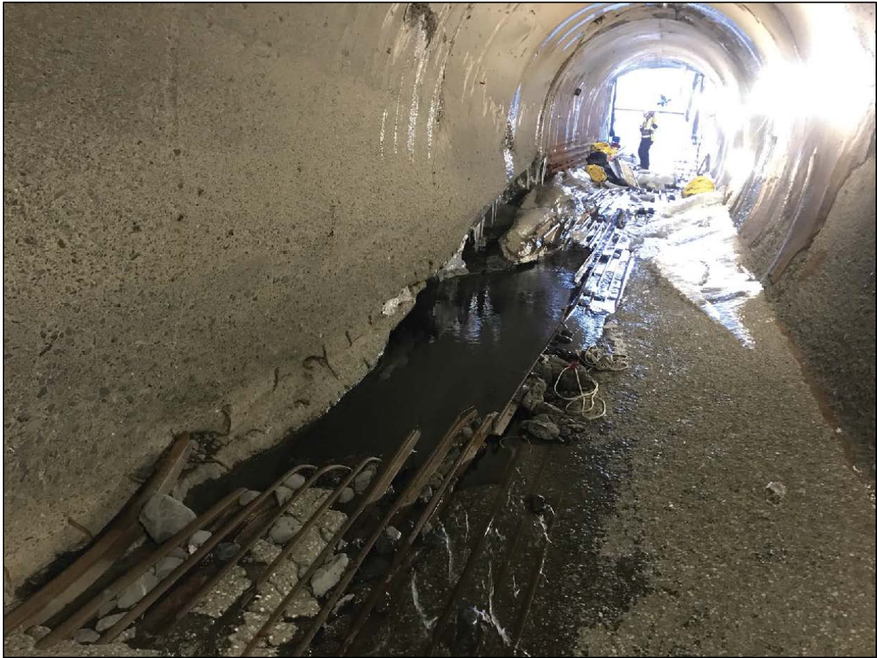
Figure 13. Large Scour Hole in Floor of Tunnel Repaired During 2017 Repairs
