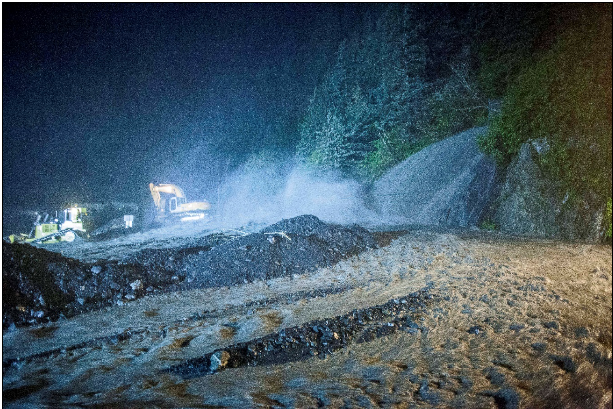
Figure 9. Heavy Equipment Removing Sediment from Tunnel Outfall during 2012 Flood
