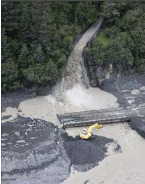
Figure 10. Lowell Creek Bridge during 2009 Flood
